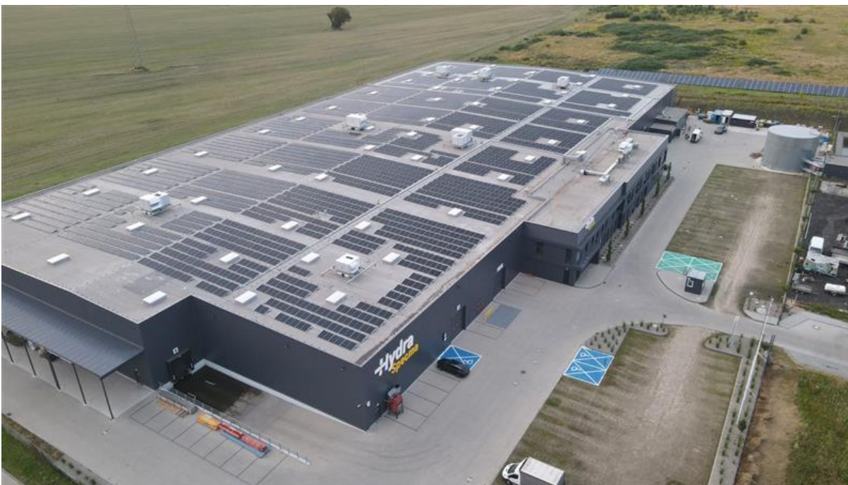
Photo – HydraSpecma new CO2-neutral factory in Stargard, Poland.
